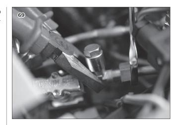
7 Utilizing two 17 mm wrenches, disconnect from the valve the incoming copper pipe from the boiler.
