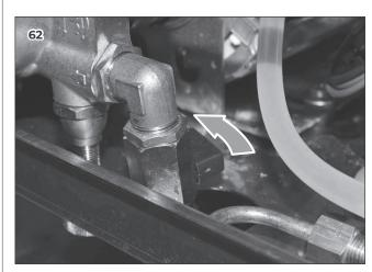
4 Utilizing two 17 mm wrenches, disconnect the incoming and outgoing copper pipes from the valve.
